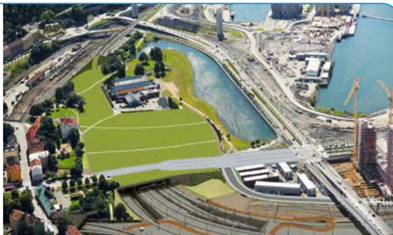
After: Rail constructions and Oslo Medieval Park in 2021
